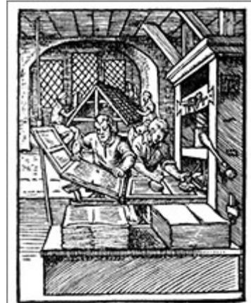
Gutenberg-style printing press from 1568. Such presses could make 240 prints per hour.
